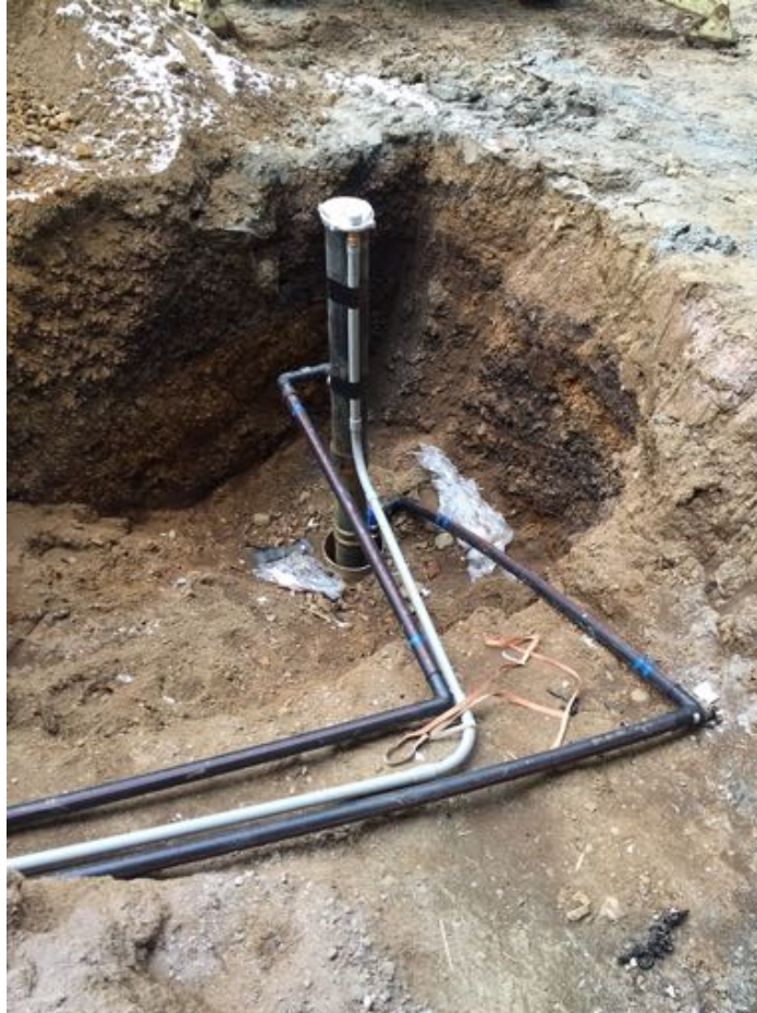
2 – 1000' deep Standing Column ® Geothermal Wells ALL heating/cooling and domestic hot water for ALL 25 apartments
