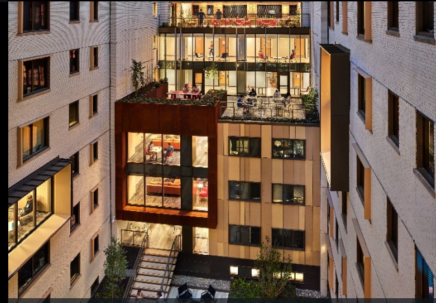
GWU Thurston Hall Renovation
