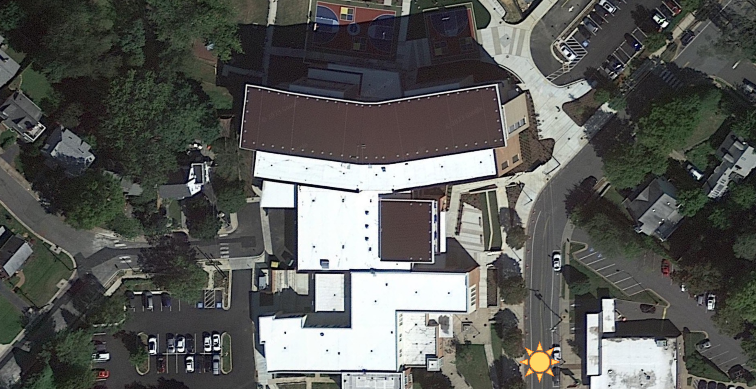
Clean Roofs: no MEP equipment and stormwater on the ground
