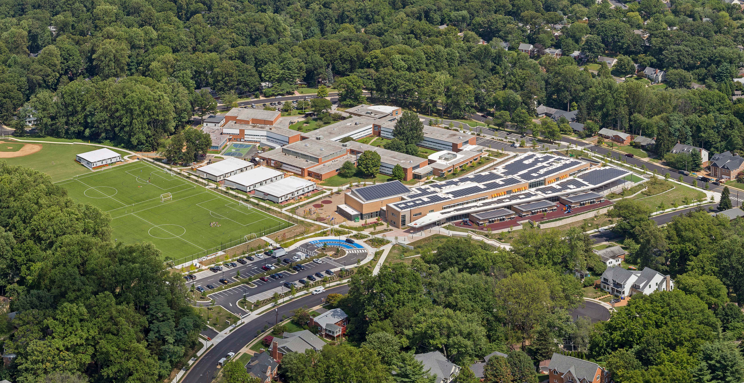
Discovery ES – first net-zero-energy building in Mid-Atlantic
